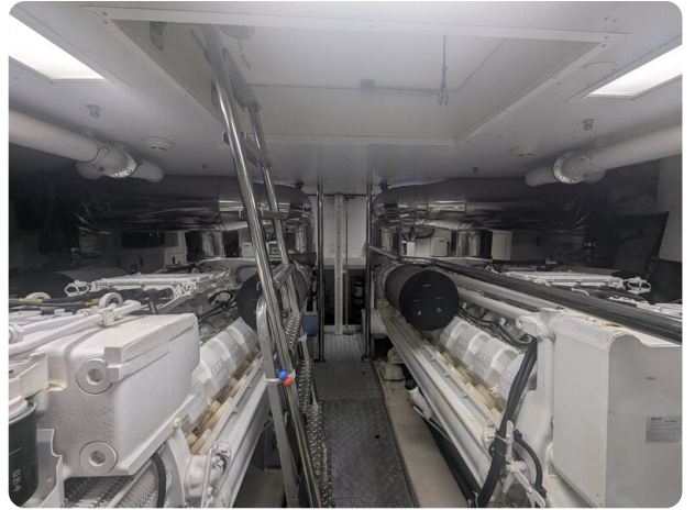
Riva 85 Opera engine room
