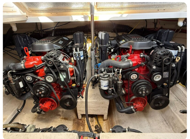
CHAPARRAL SIGNATURE 310 Engine room
